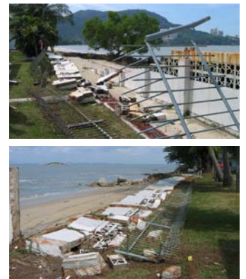
Dalat's broken seawall protected lower-campus classrooms. Construction has already begun on a new wall.
